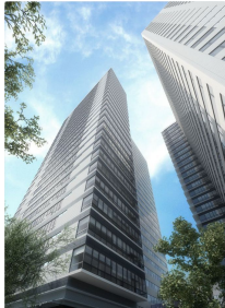
Vista exterior del edificio Lower view of the building
